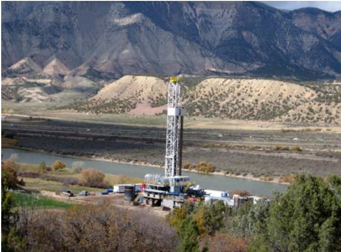
Figure 3. Helmerich & Payne rig drilling for Williams Company.
